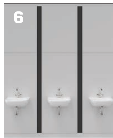
6. Install the remaining cladding.
